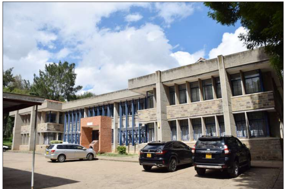
The front view of the Faculty of Arts and Social Sciences building at the Main Campus, Njoro, seen from the parking lot
