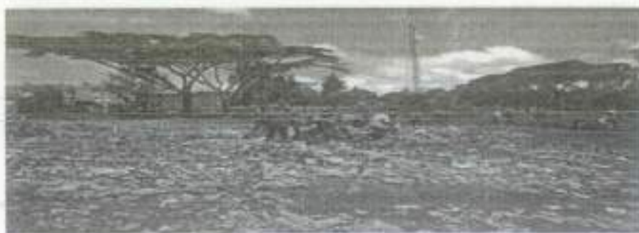
Part 1 Dump site as at 10 th May 2015 before bulldozer descended on it.
